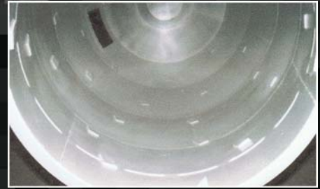
Concrete drum coated with Metallic Polymer
